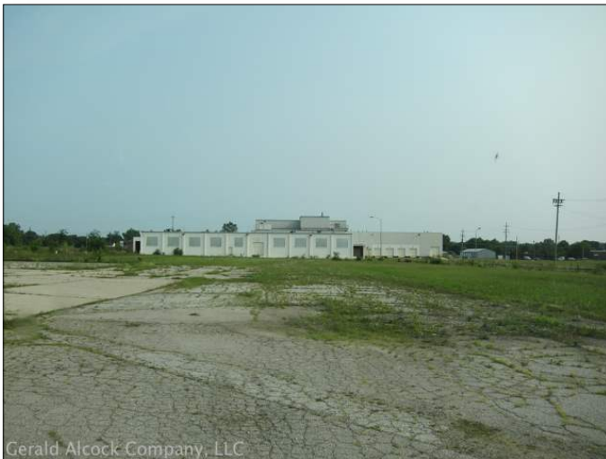
View of Site; Facing North
