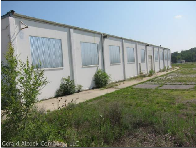
Rear or South Elevation; Facing East
