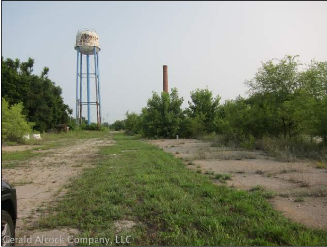
View of Site; Facing North
