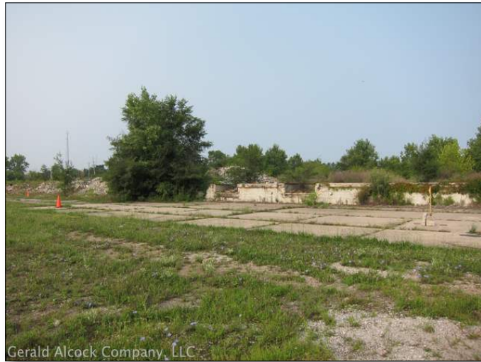
View of Site including Slab of Demolished Building; Facing East
