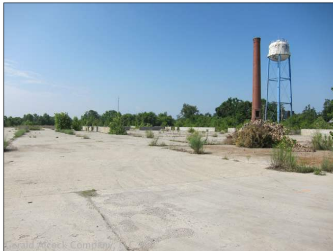
View of Site including Slab of Demolished Building; Facing South
