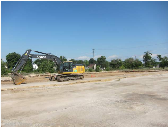
View of Site; Facing North
