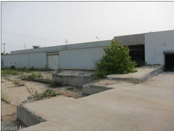
Partial Side or East Elevation; Facing West
