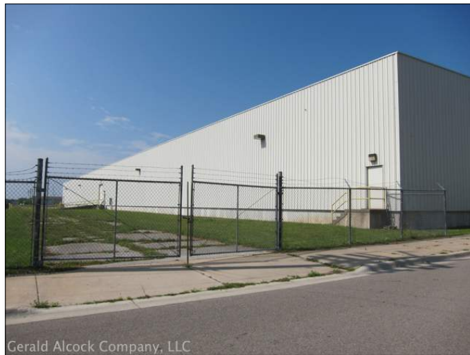
Side or East Elevation; Facing South
