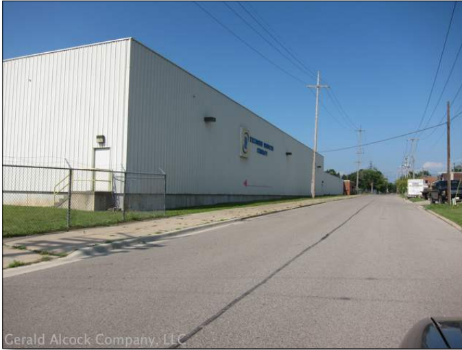
Front or North Elevation; Facing West
